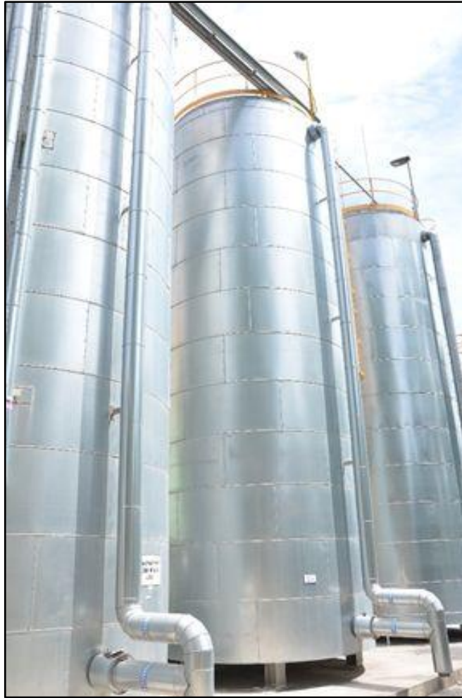
Figure 16 Storage of urea for denitrification in Turów power plant
