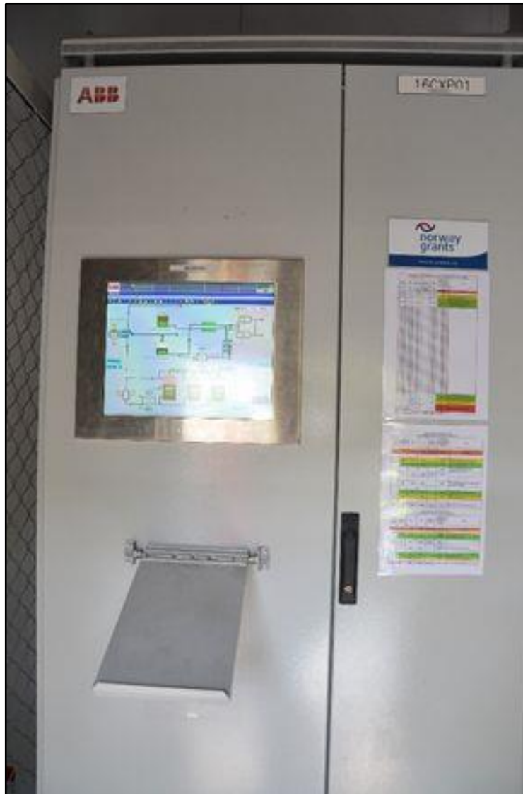
Figure 15 Urea denitrification control unit in Turów power plant
