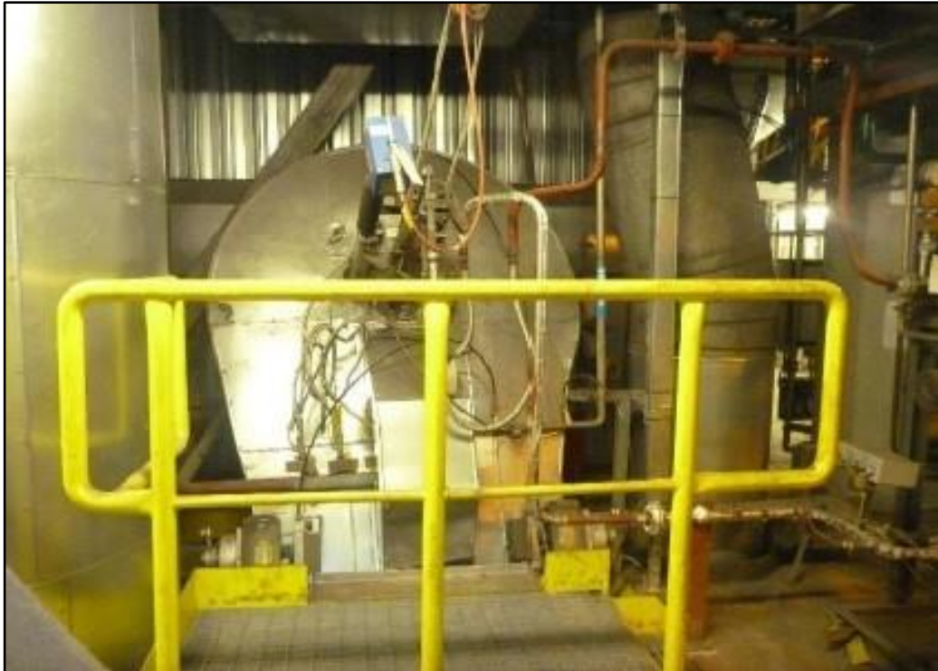
Figure 19: Reconstruction of boiler K1 in order to adapt to the combustion of biomass in Siekierki
